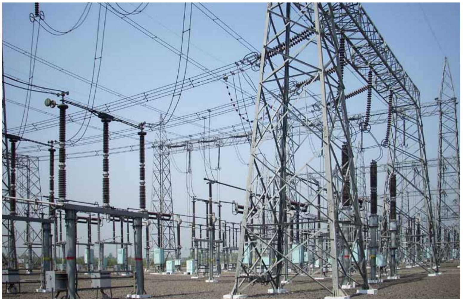
Primary injection test equipment is much easier to use than it used to be
